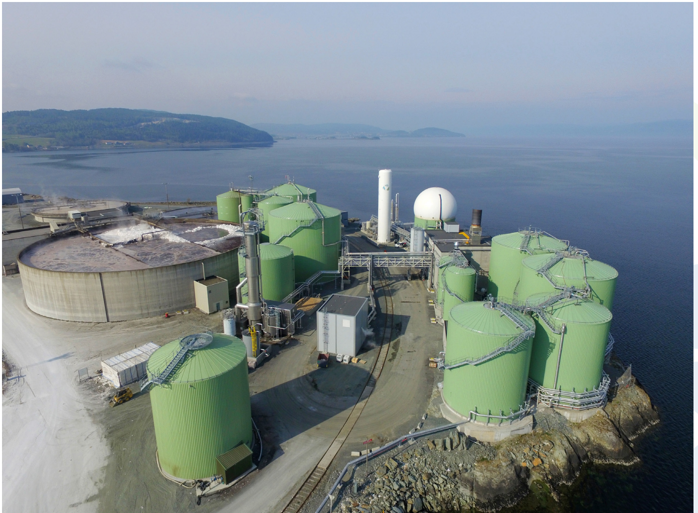
Example of an evaporator system for purification of process water with a capacity of up to 200 m3/hour and an energy consumption from 8kWh/m3.
